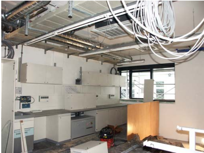
The lab in April: >> under construction.<<
